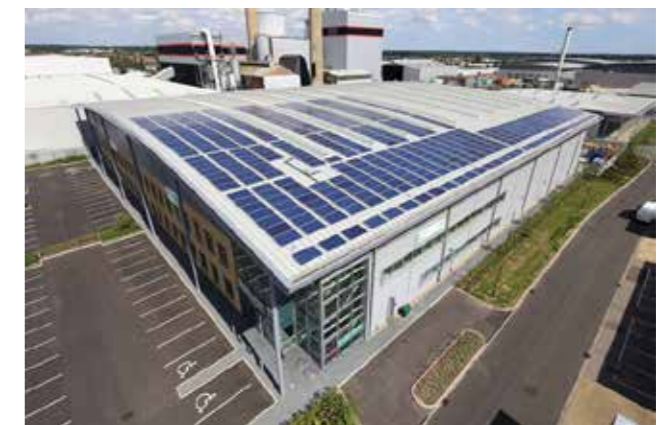
Fig. 39: Photo voltaic panels located on roof
